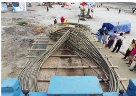
Figure 1: Cable Installation toward Beach Manhole
