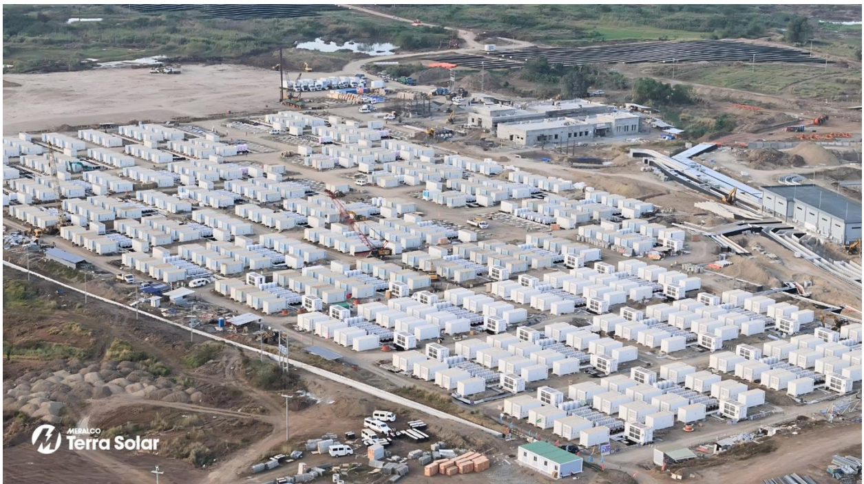
The MTerra Solar project is the world's largest integrated solar PV and battery facility. Once fully completed, it will deliver 3,500 MWp of solar PV capacity paired with 4,500 MWh of BESS.
